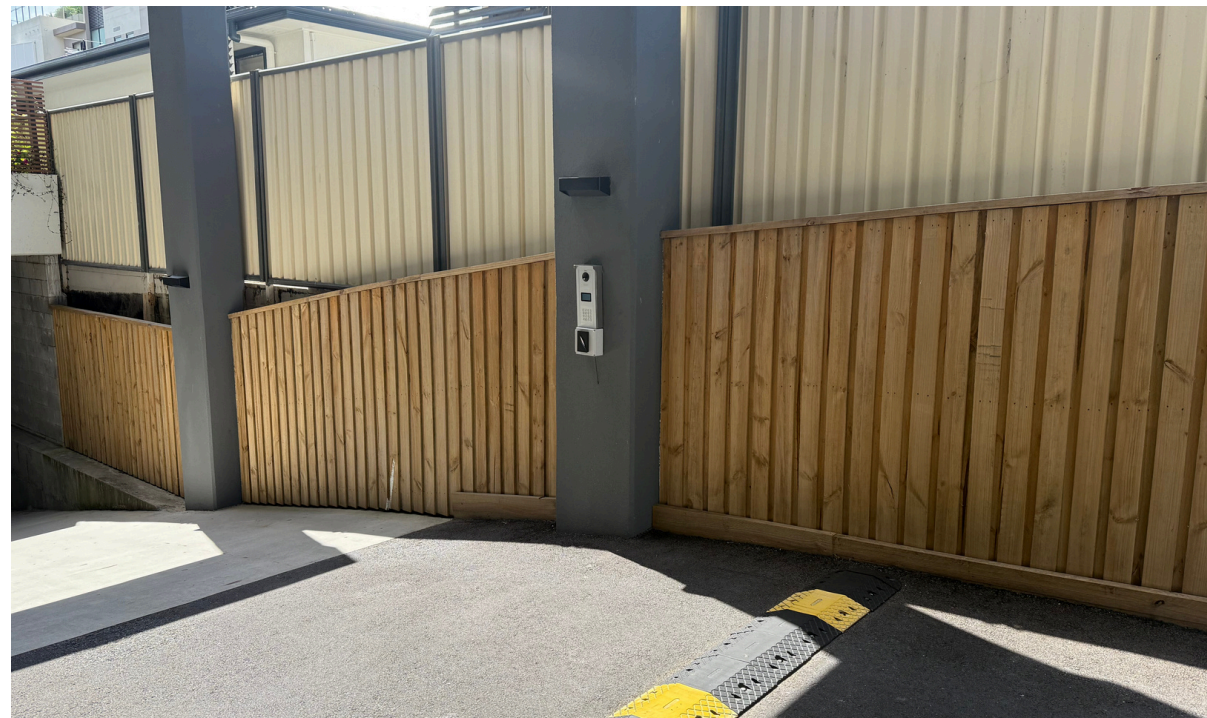
Acoustic fence with 65 x 65 gal posts at rear
