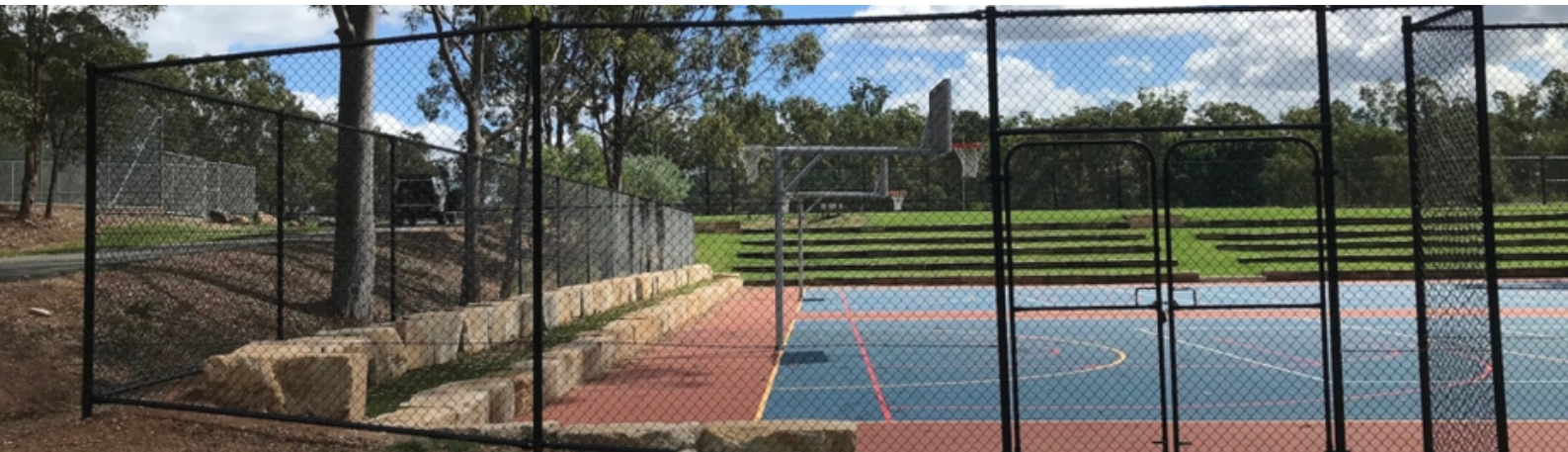
3000mm high black chainwire fencing for Basketball court
