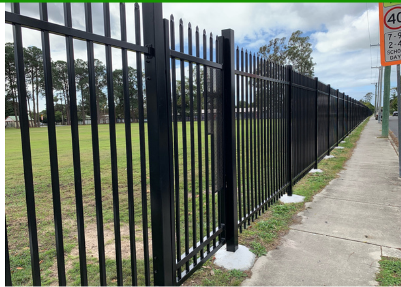
DETE Spec 2100mm high spear top fencing and gate at northern bayside state school
