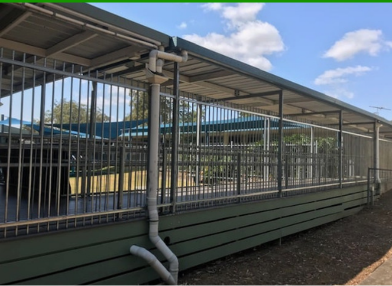
1800mm high galvanised steel panels for a northside Special School
