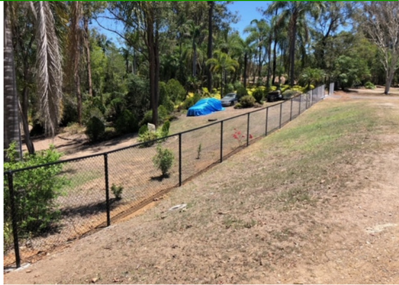
1500mm high black chainwire fencing across front boundary of Acreage property.
