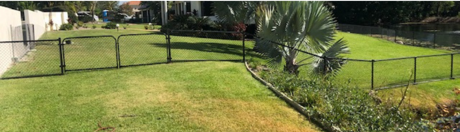
900mm high black chainwire fencing on rural residential property to section off house.
