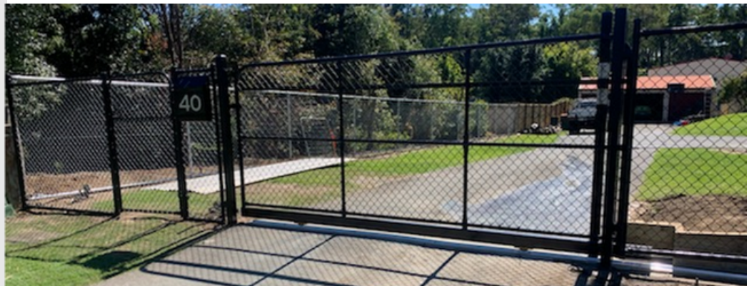
1500mm high black chainwire fencing and sliding gate.
