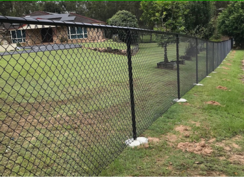
1500mm high black chainwire fencing with top rail.
