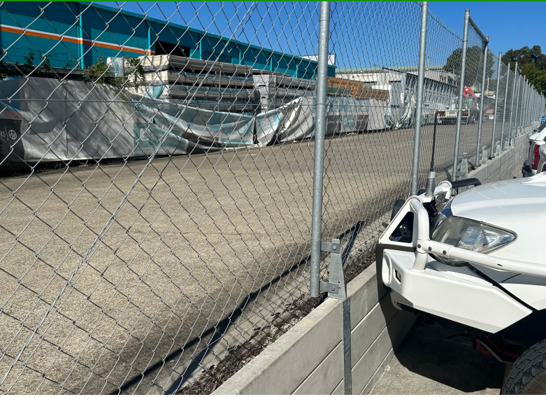
Chainwire fence on top of concrete retaining wall.
