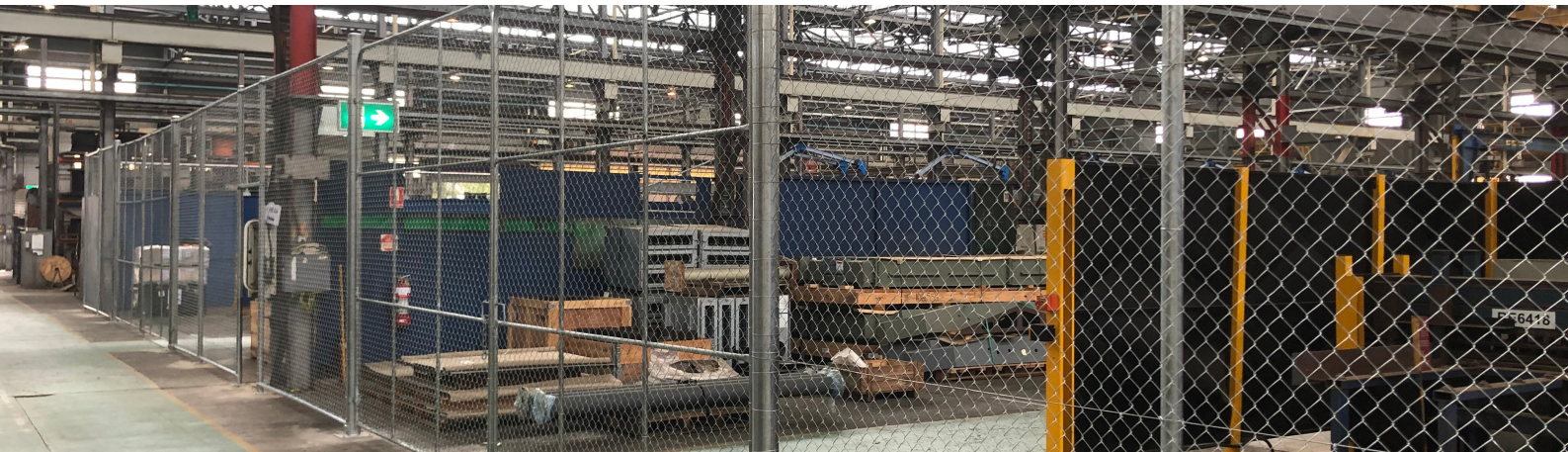
Chainwire Fencing enclosure for a supermarket distribution centre.
