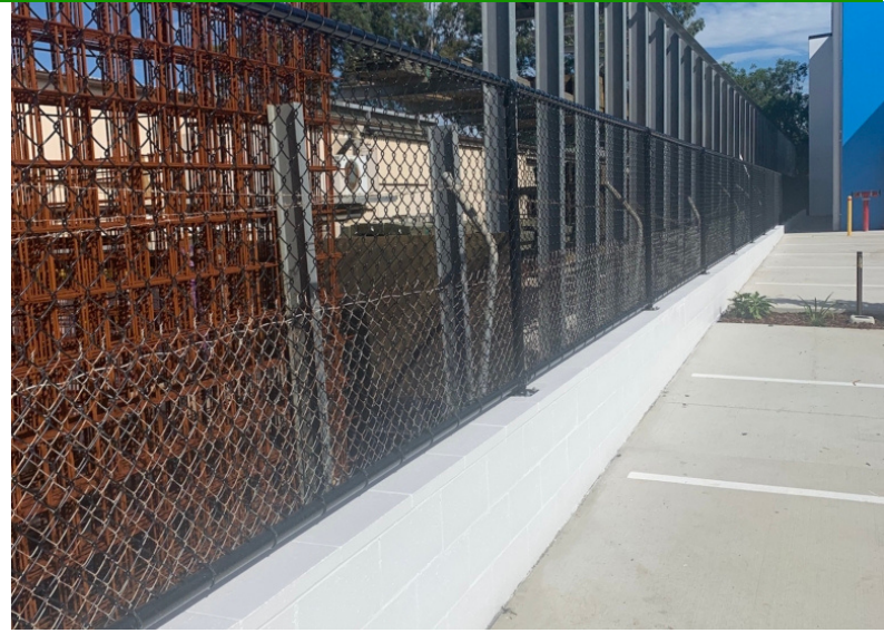
1200mm high black chainwire fencing mounted onto a block wall.
