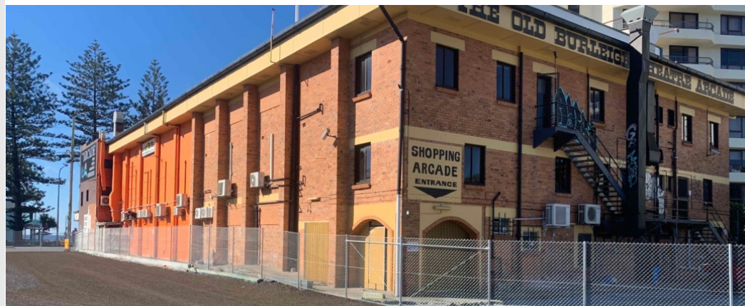
1800mm high galvanised chainwire fencing.
