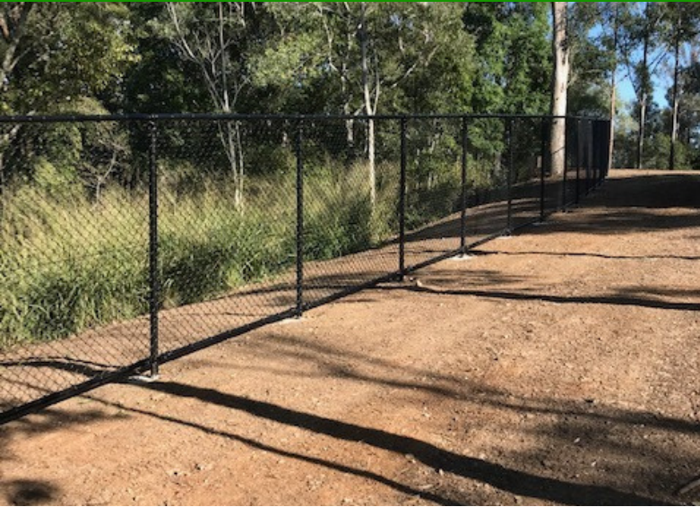
1800mm high black chainwire with top and bottom rail – Samford.
