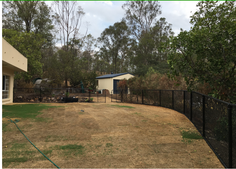
1200mm high black chainwire with top and bottom rail – Dayboro.
