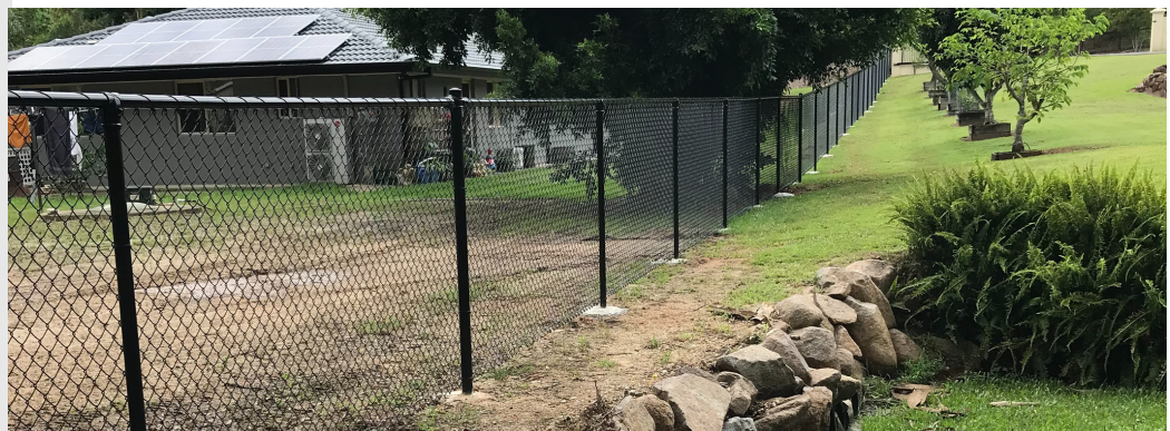
1500mm high Black Chainwire with top rail – Eatons Hill.
