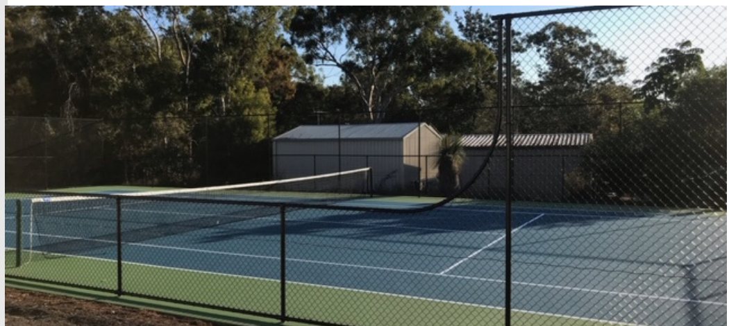
3000mm high transitioning down to 1200mm high with curved rail for a Tennis Court.
