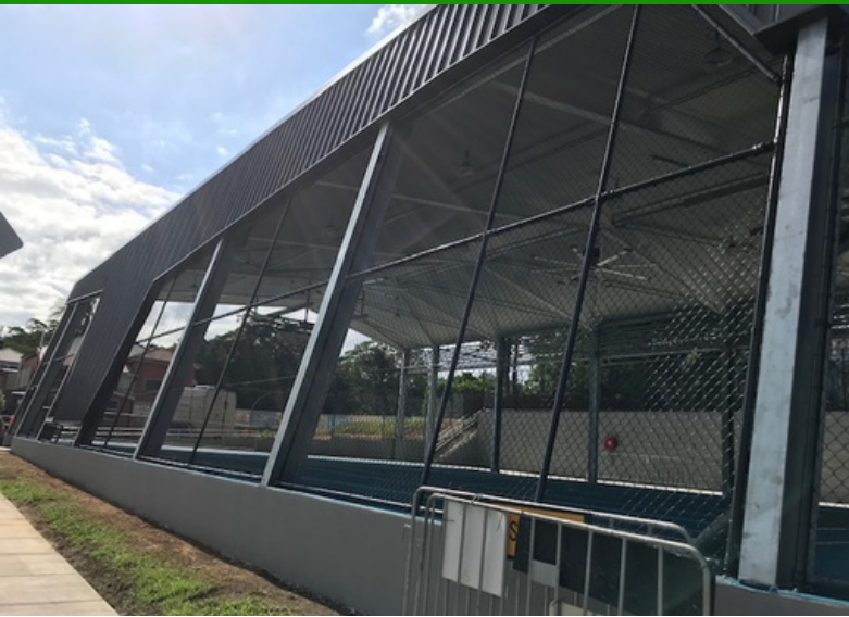
Chainwire infills on the side of Multipurpose Courts at a Primary School.
