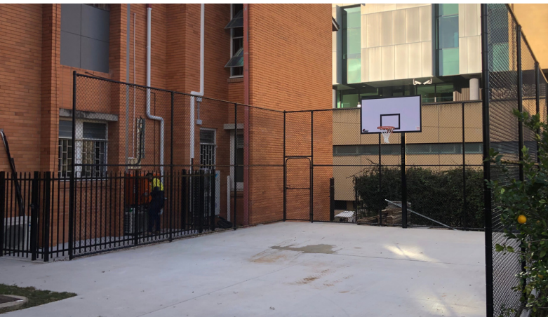
Chainwire infills on the side of Multipurpose Courts at a Primary School.
