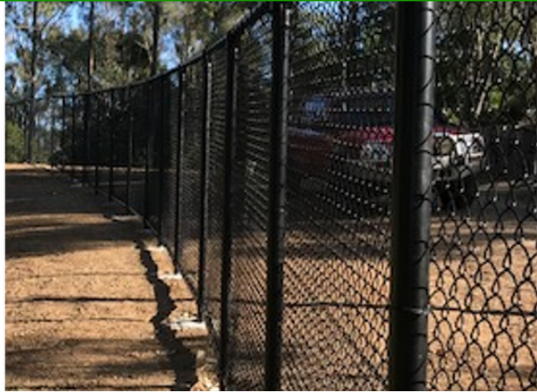
1800mm high Black Chainwire fence with top and bottom rail
