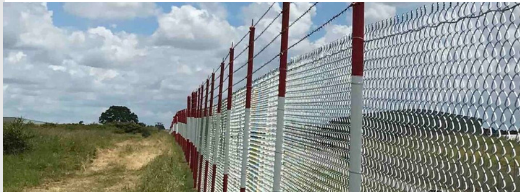
1800mm high chainwire security fencing with 3 strands of barbed wire on top for an airport
