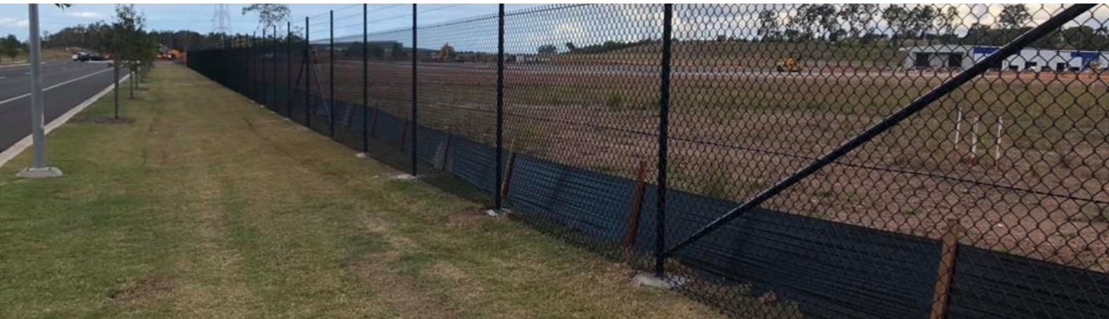
1800mm high black chainwire fence with heavy duty chainwire and 3 strands of barbed wire on top
